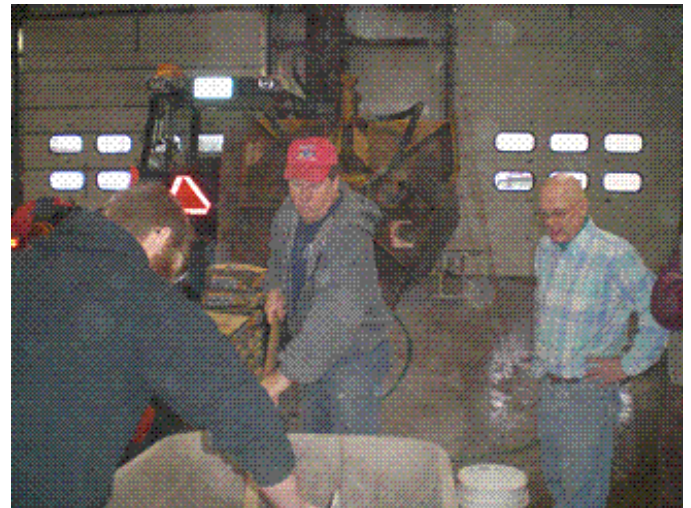
The concrete was mixed by hand.
